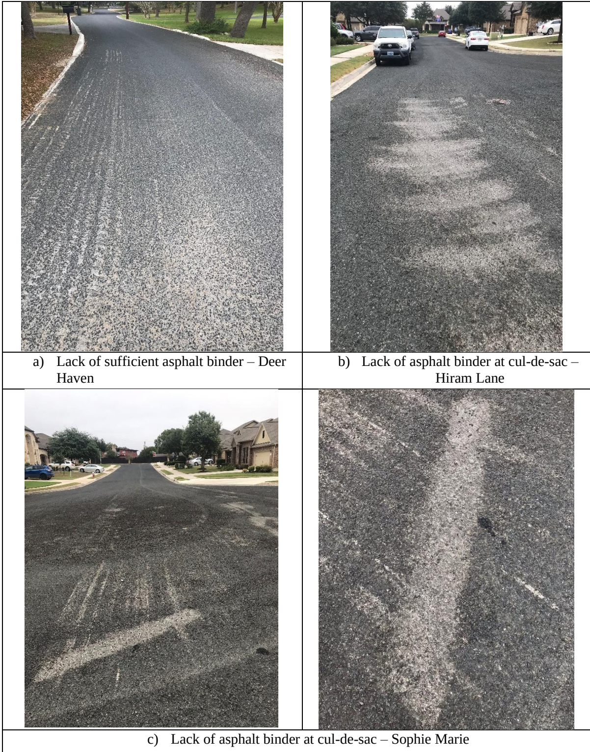
Figure 3- Exposed pavement surfaces on chip seal projects
